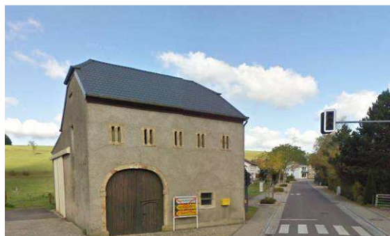
Hangar agricole - Route de Luxembourg
